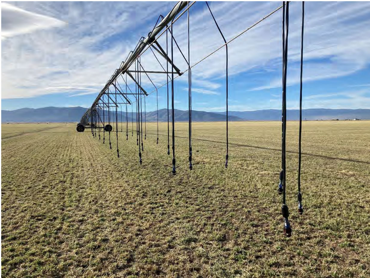
Photograph of Installed LEPA Sprinklers on Roberti Pivot #13
