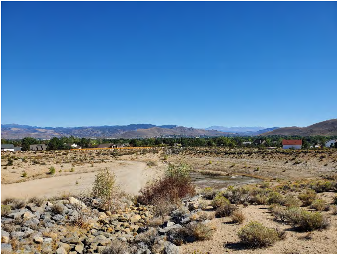
Photograph 4.1 – Ground view of an infiltration basin on the Vice Canyon alluvial fan
