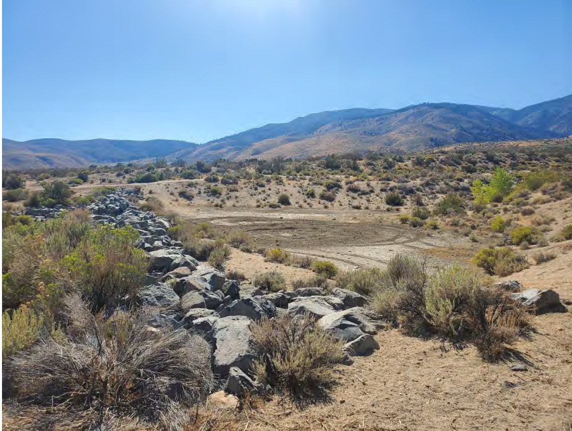
Photograph 4.2 – Ground view of an infiltration basin on the Vicee Canyon alluvial fan
