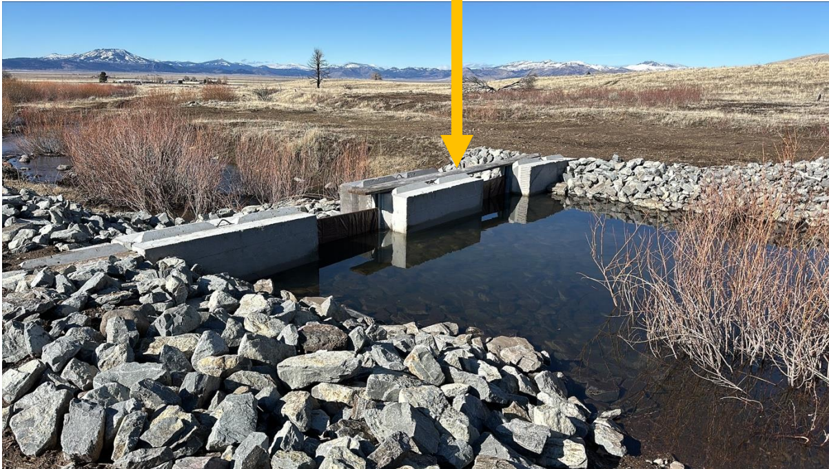
Check Dam on Staverville Creek with removable checkboards
