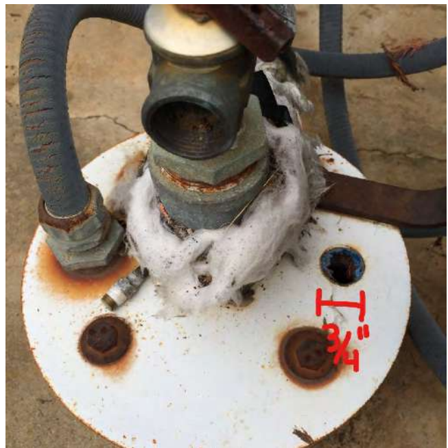
Figure 2. Example Well Opening that is 0.75 inches wide.
